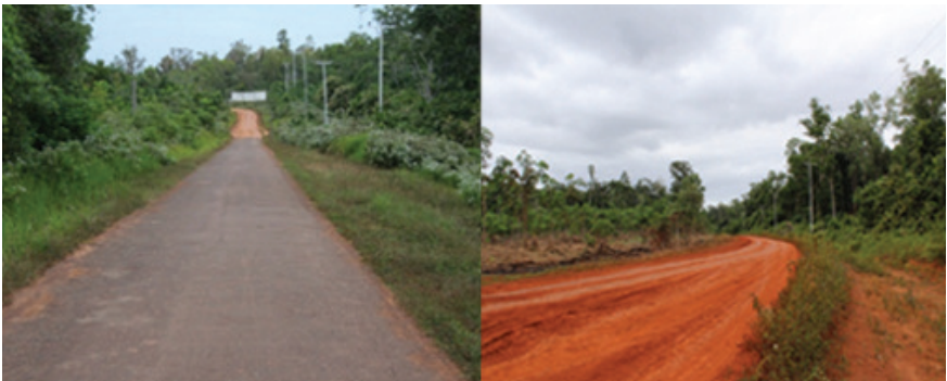
Some of the construction projects aided by the government of Merauke Regency. 26
